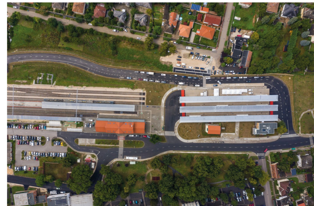
Renovated bus and train station in Esztergom
