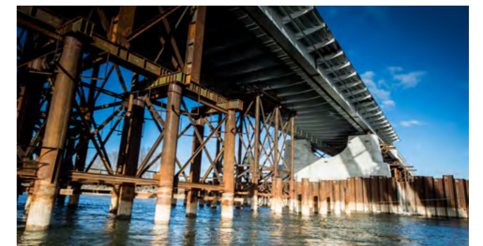
Construction of the Danube bridge in Komárom
