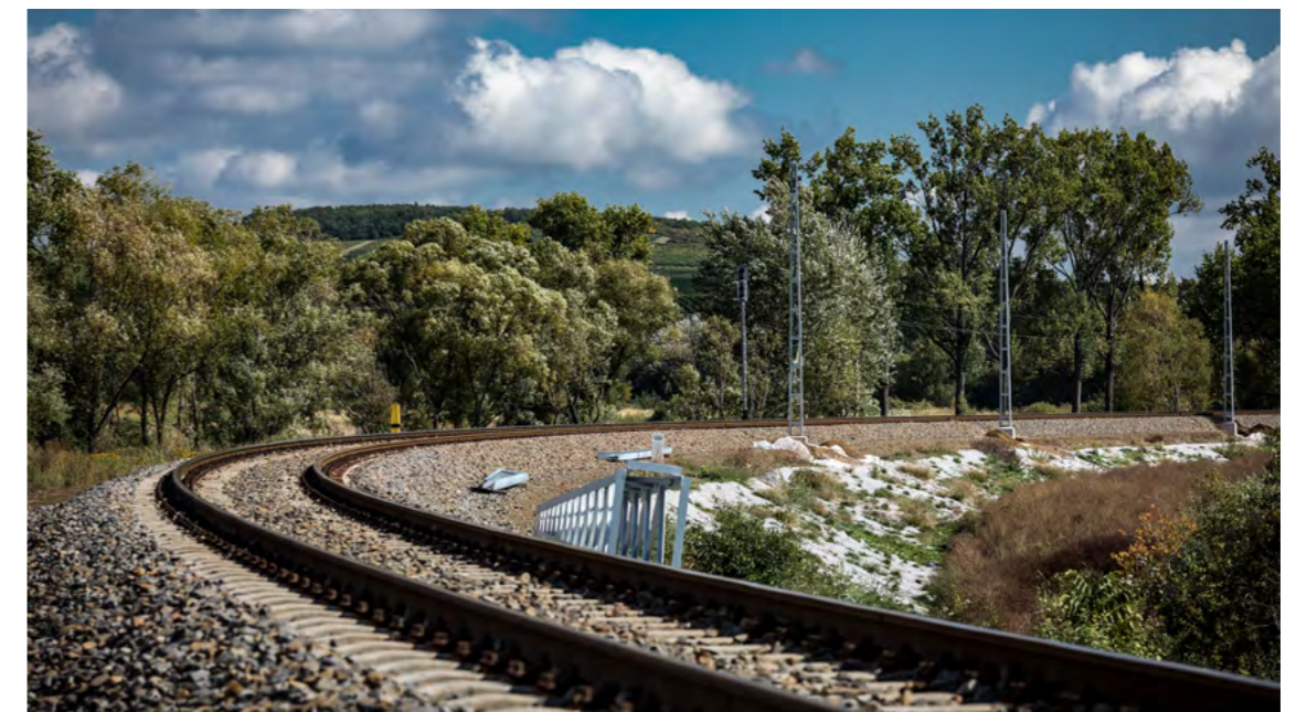
Section of the rail line between Mezőzombor and Sátoraljaújhely
