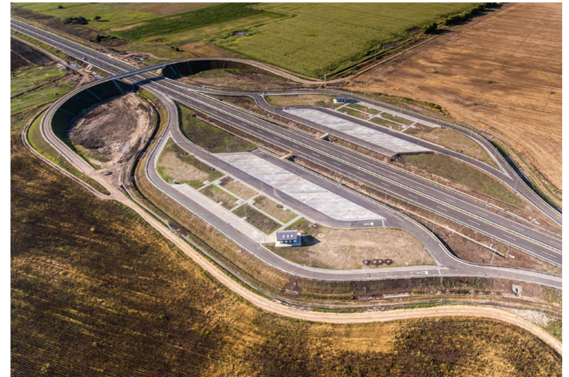
New section of the express road M44 between Tiszakürt and Kondoros
