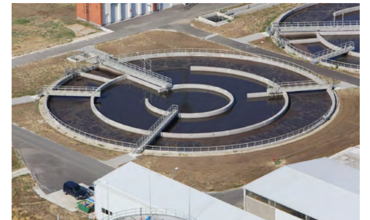
Wastewater Treatment Plant, Nagykanizsa
