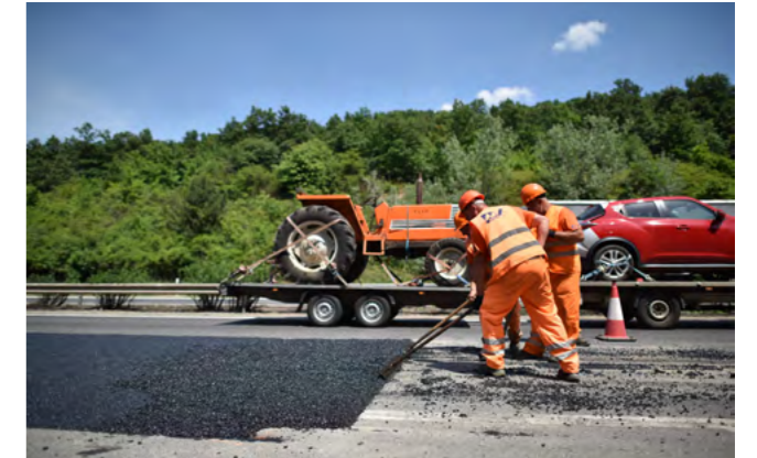
M1 motorway reconstruction
